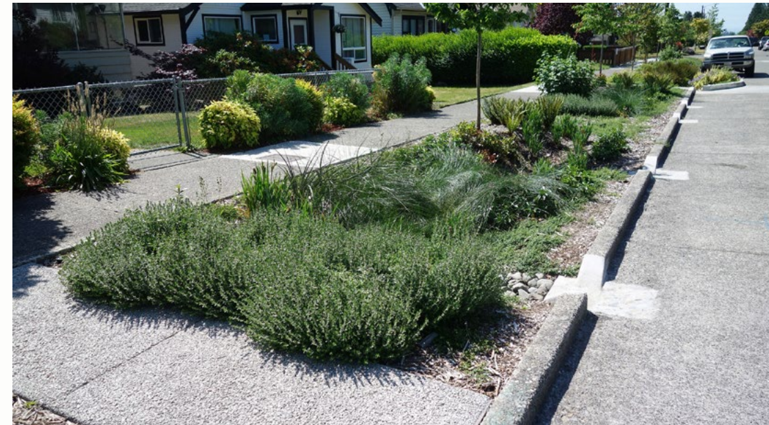
— Rain garden as part of the GSI on 34th Ave SW
