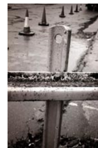
Railroad rails recycled as bollards and railings.
