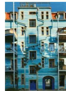
Imaginative rain downspout design with potentially sonic overtones, Germany.
