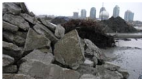
Site excavation at the 50-acre Southeast False Creek redevelopment site showing the stock piled rubble, a possible recyclable resource.
