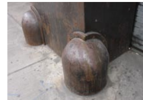
Cast iron wheel guards, typically flanking truck portals into buildings, an architectural detail which reinforces the industrial identity and suggests entry or gateway.
