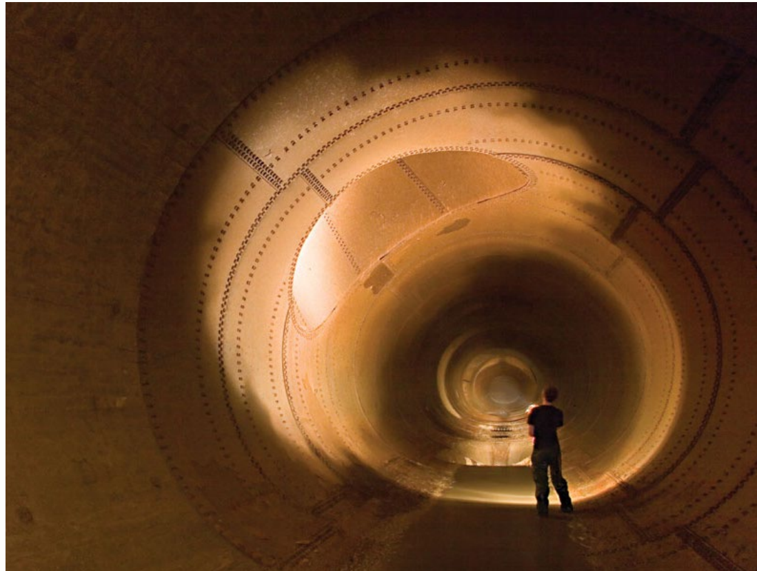
— Conveyance pipe, Toronto, Canada. Photo by Michael Cook
