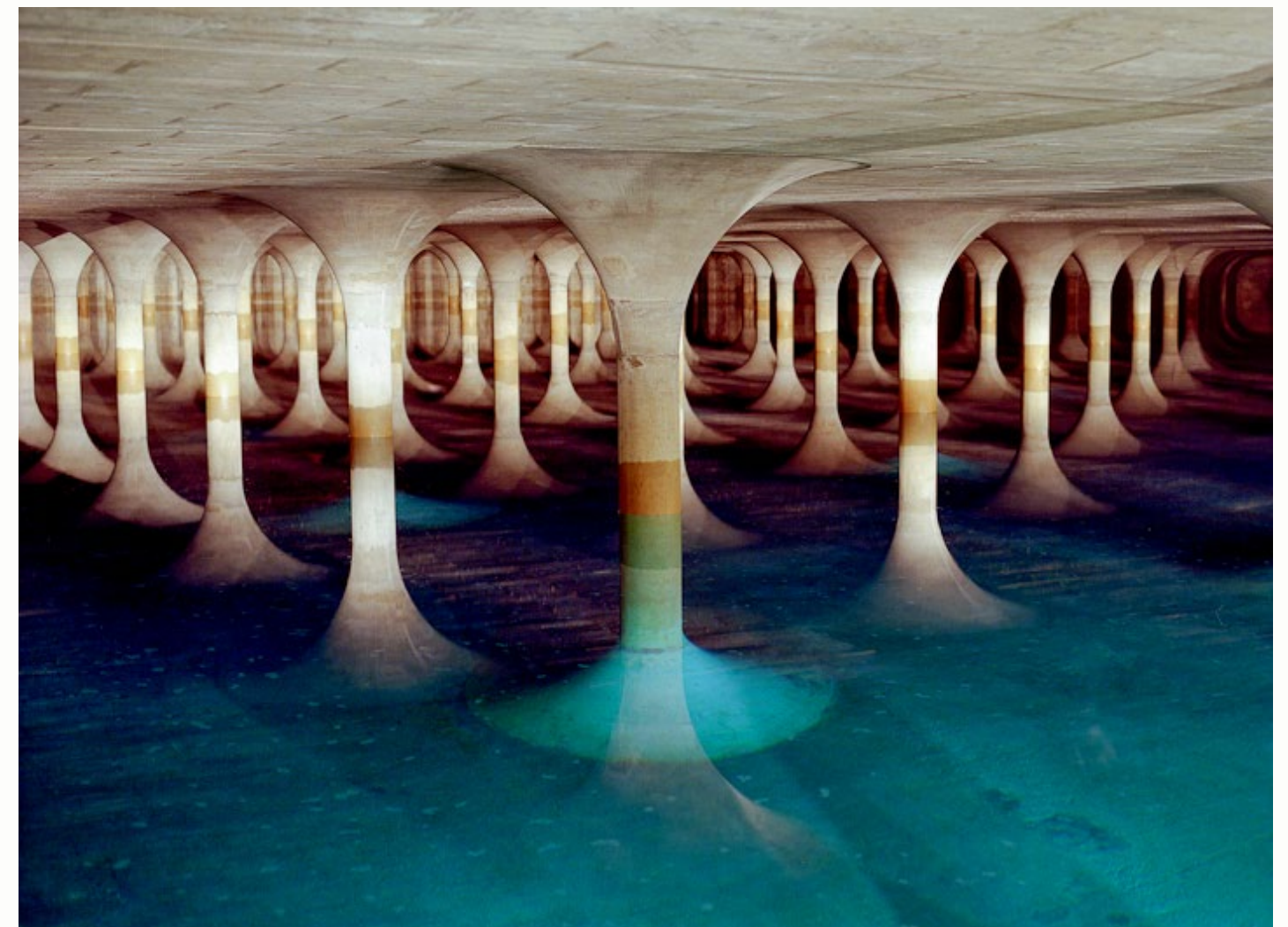
– Drinking water reservoir in Forstenried Park, Munich, Germany Photo by Peter Neusser
