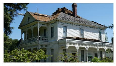
In the process of tearing off old shingles and installing new, cedar shingles, original skipjack boards were exposed on the east side of the Neely Mansion roof, 2023. Photo: Neely Mansion Association, Linda Van Nest
