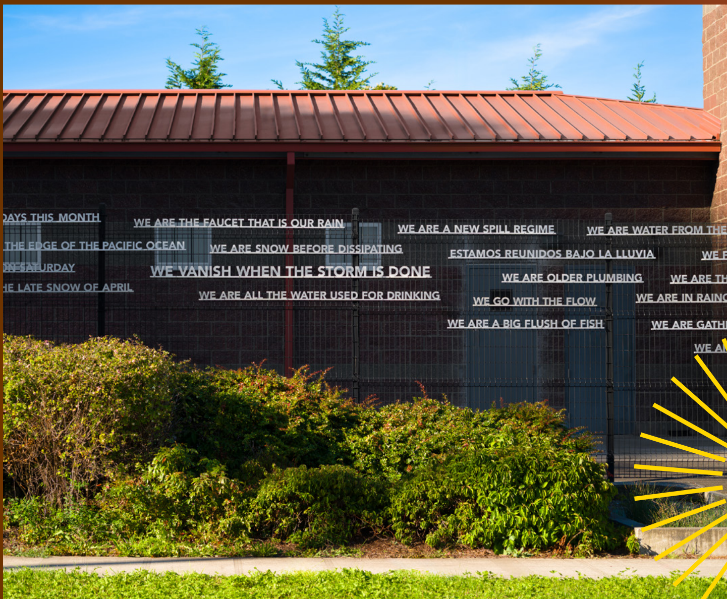
AREA C Projects. Water Log (detail), 2025. Aluminum. King County Public Art Collection. Rainer Valley Wet Weather Storage, Seattle, WA. Photo: joefreemanjunior.com
